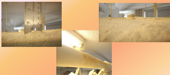
Result of Improper Dust Collection Systems
